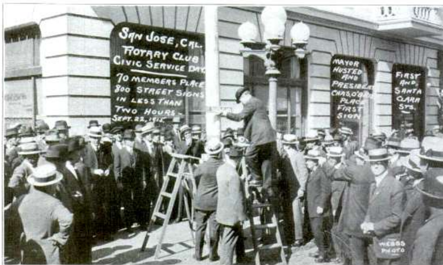
Putting up the first street sign; Mayor Husted on the ladder; President O'Brien of the San Jose Rotary Club in straw hat tacking on the lower sign.
